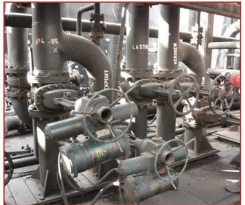
Complex manifold, some motorised valves, most manual.
