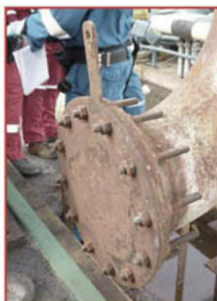
Pump Discharge – plate used instead of blind flange
