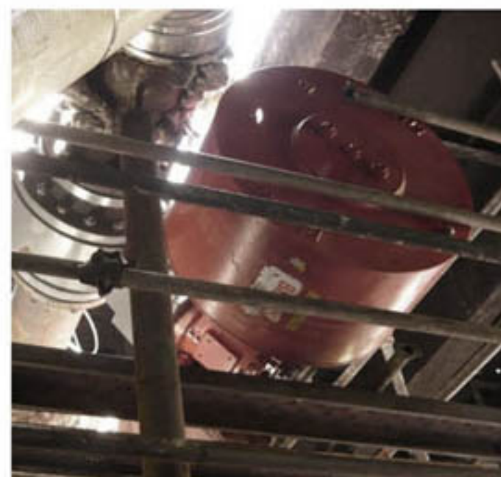
328 valves originally identified. Scope now reduced to 21, using PDVSA 1997 criteria of 25m 3 inventory. Another ~20 will be needed. Scope now includes Overhead drum sour water draw valves. 5 valves installed at CD-4. Had this been implemented sooner, the consequences of the February 2012 CD4 fire would have been significantly reduced. (See pictures below). Legacy issues – Cardon EIVs are fail-safe pneumatic, those at Amuay are electrical drive.
