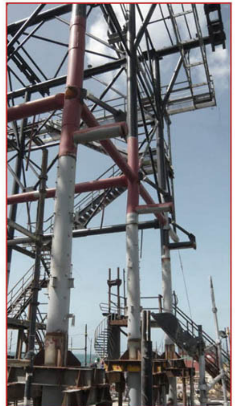
Substantial sections of Upper Hose Handling Structure replaced.
