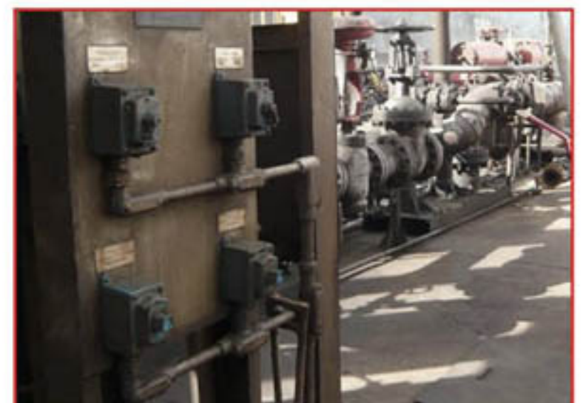
Emergency Isolation valve, failsafe, (air to open, spring to close) some confusion about tag nº, fireproof cover not replaced, actuation from local switch only.
