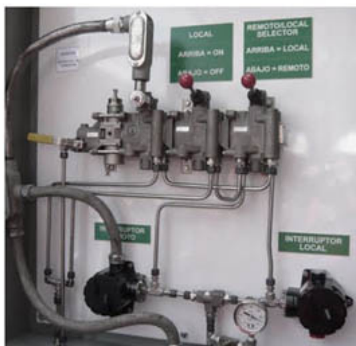
328 valves originally identified. Scope now reduced to 21, using PDVSA 1997 criteria of 25m 3 inventory. Another ~20 will be needed. Scope now includes Overhead drum sour water draw valves. 5 valves installed at CD-4. Had this been implemented sooner, the consequences of the February 2012 CD4 fire would have been significantly reduced. (See pictures below). Legacy issues – Cardon EIVs are fail-safe pneumatic, those at Amuay are electrical drive.
