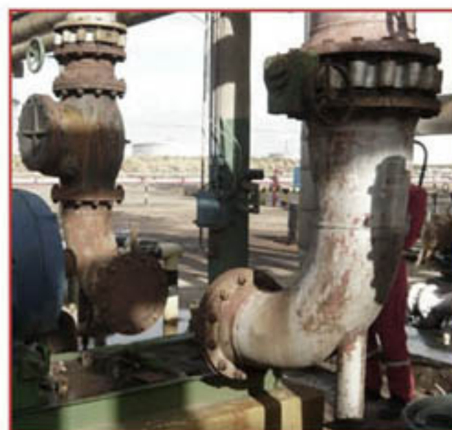
Same pump – valves not tagged or locked.
