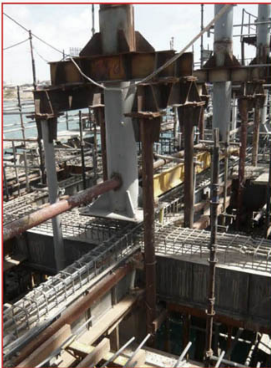
Substantial sections of Upper Hose Handling Structure replaced.
