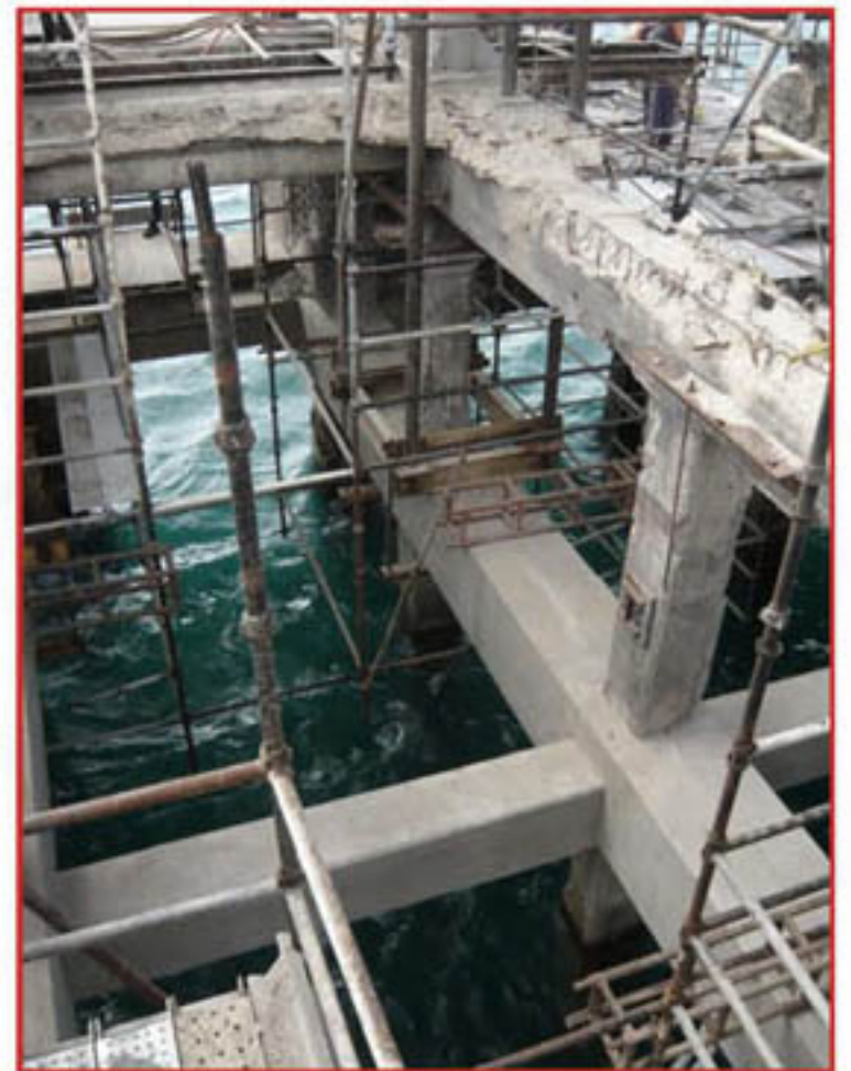
Under-deck structure extensively replaced
