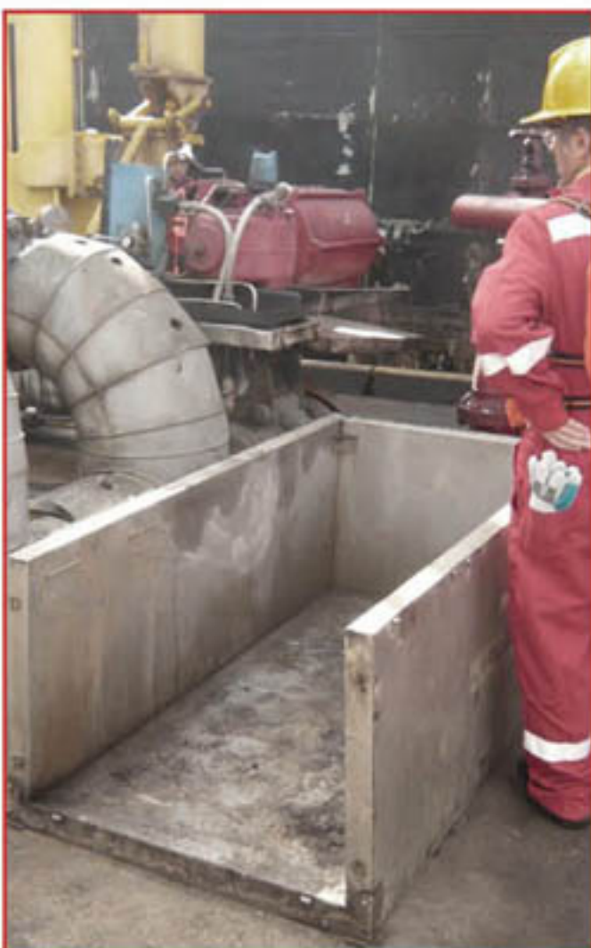
Emergency Isolation valve, failsafe, (air to open, spring to close) some confusion about tag nº, fireproof cover not replaced, actuation from local switch only.
