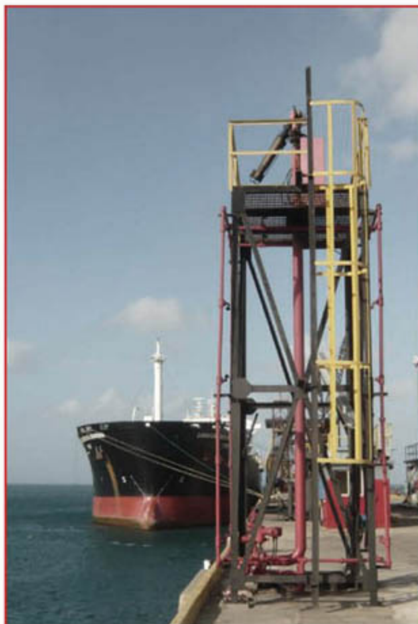
Remote operated steerable elevated foam/water monitor.
