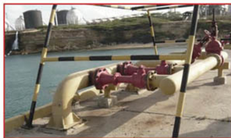
Foam solution manifolds and air venturis for under-deck foam curtain
